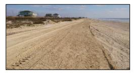
**GIWW-Rollover Bay Reach Beach Nourishment with Beneficial Use of Dredged Material** (BMMP maintenance project) – Beach nourishment project beneficially utilizing approximately 173,000 cubic yards of dredged material, from the U.S. Army Corps of Engineers Fall 2013 maintenance dredging of the GIWW
