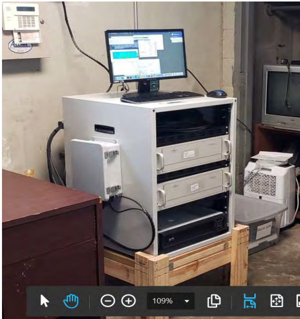
Figure 13 Rack mounted SeaSonde electronics inside Moses Lake Tide Gate Control Building
