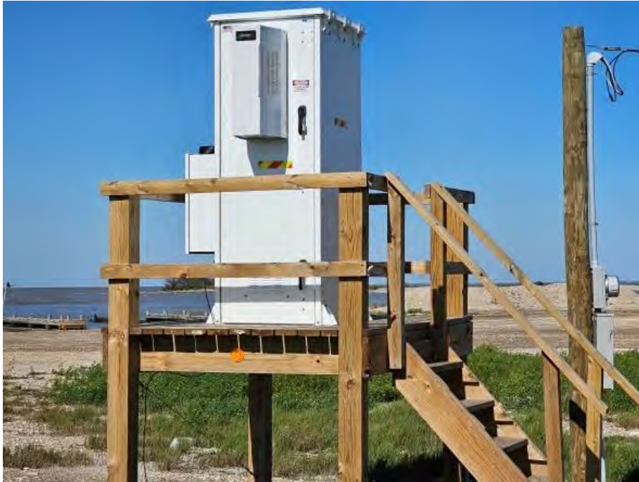
Figure 16 Climate controlled enclosure on elevated deck at Smith Point. Power for statin provided through the meter to the right side of enclosure
