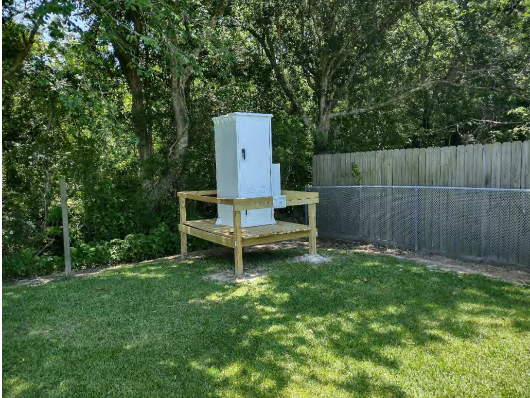
Figure 14 View of climate-controlled enclosure at McCollum Park
